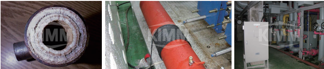
〈 Existing Pipe Scale and Newly Developed and Installed Scale Removal Device 〉
