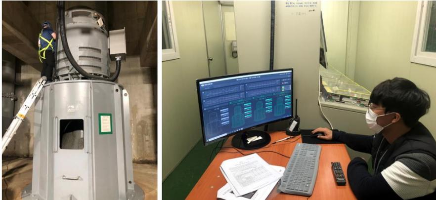
Photo description: The AI-based predictive diagnosis technology developed by Dr. Kyung Ho Sun's research team at the Dept. of System Dynamics, KIMM, is being used to diagnose the condition of the drain pump at the dry dock of the ROK Navy's maintenance depot.
