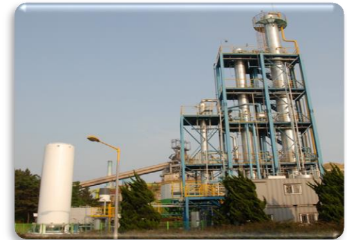
CO 2 Capture Pilot Plant (10 t-CO 2 /d) @ POSCO-Pohang Works
